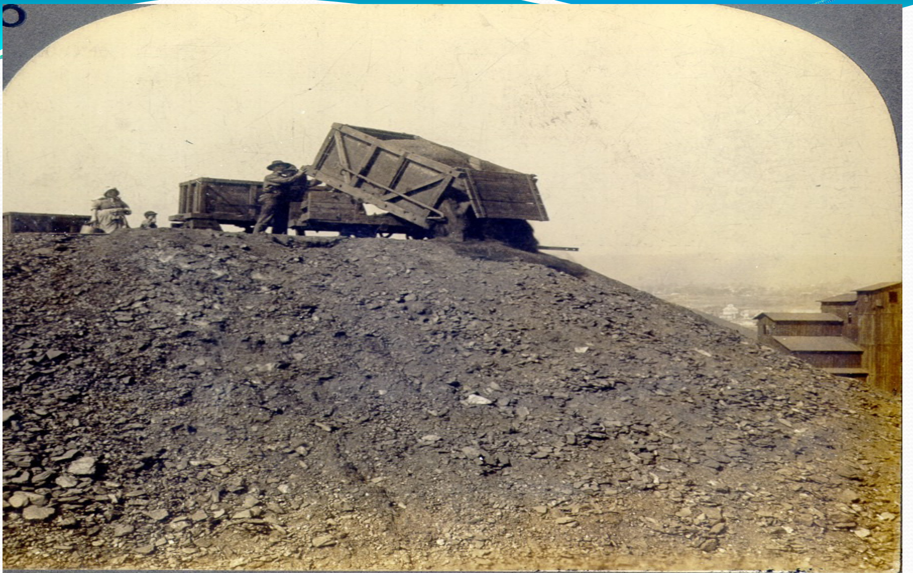
7069—Dumping Culm, Slate Pile, Anthracite Coal Minin Scranton, Pa., U. S. A.
